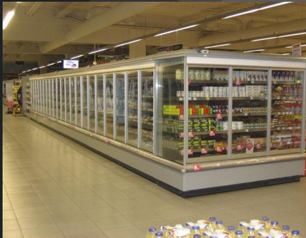
**EcoPlus** solution is made of **PVC frame** doors with double glass panel for positive temperature cabinets.
