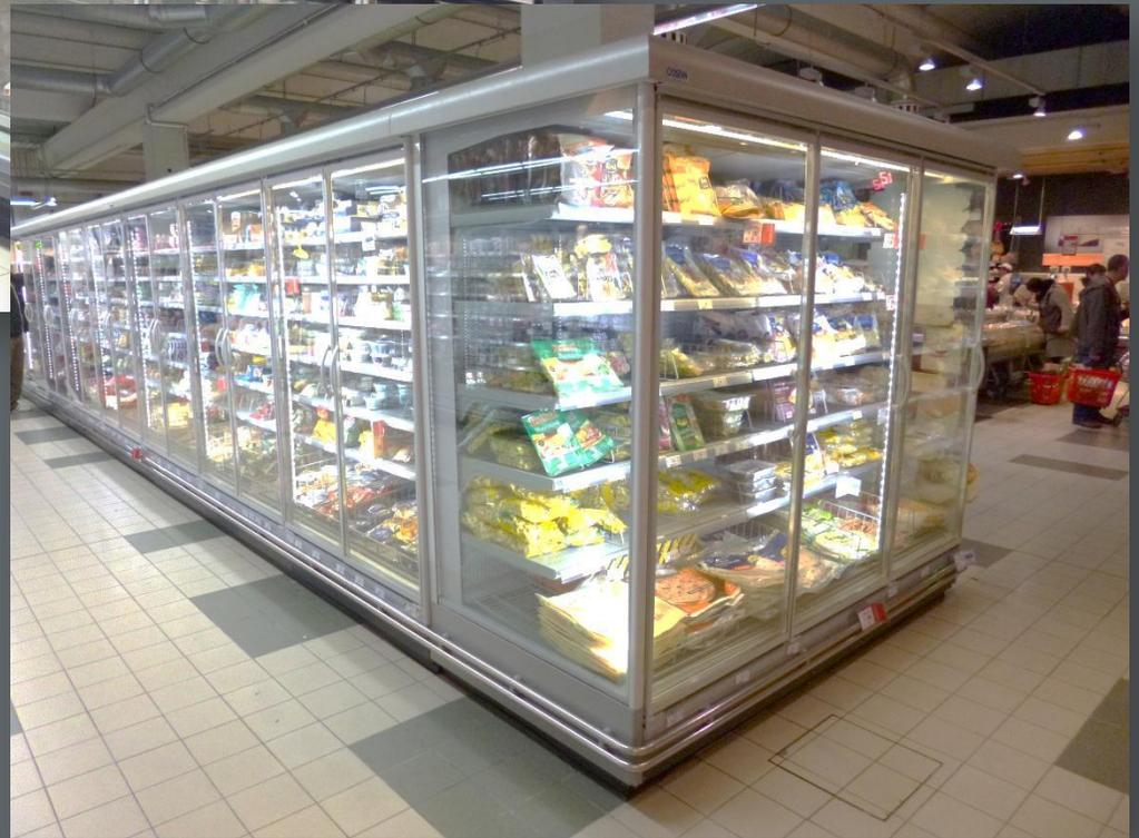
**Mono** solution is made of **single glass doors** without vertical profiles.
