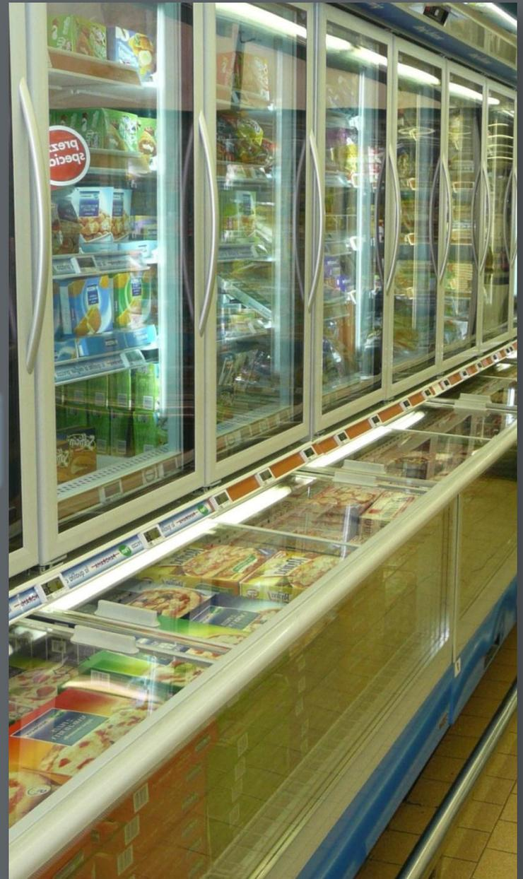
**Plug-in** solution is made of **plastic frame** with single glass **sliding lids** for plug-in islands .
