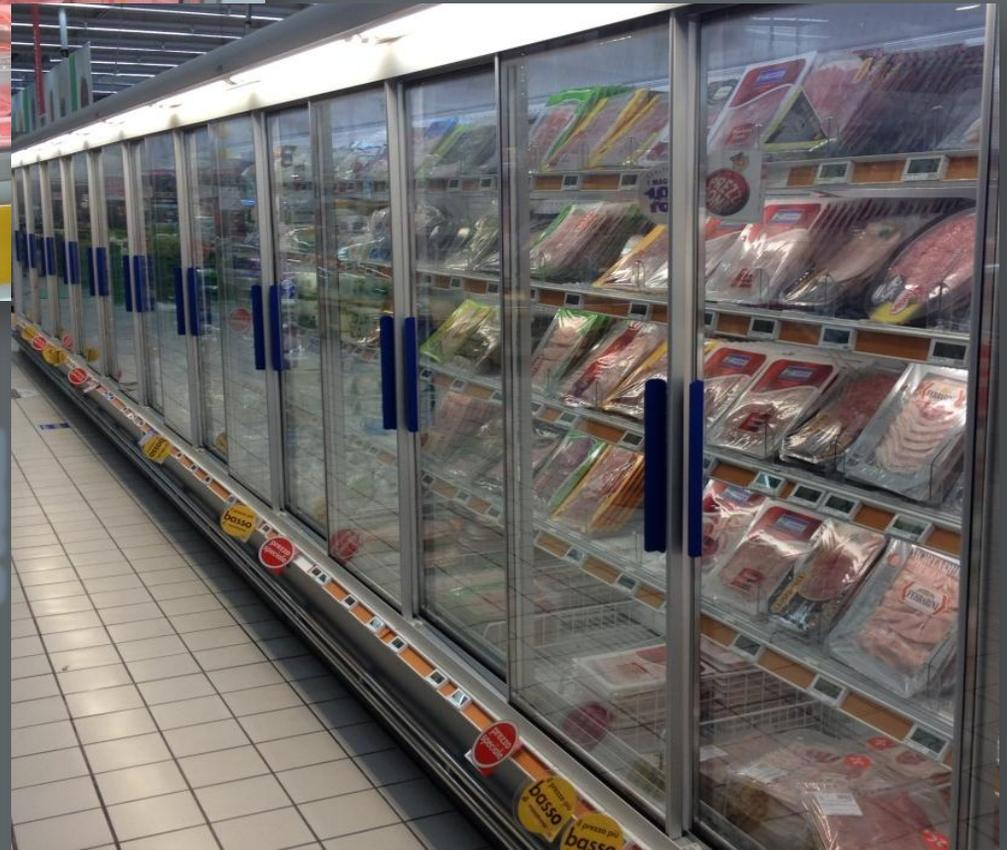
**Slide** solution is made of **single curved glass doors** with slide motion.
